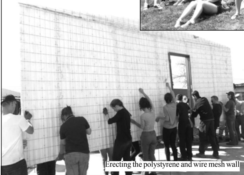
Erecting the polystyrene and wire mesh wall
