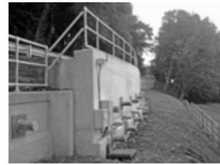
Fig. 2 West End of new retaining wall with tension pile anchorages visible in the foreground
