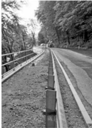
Fig. 1 Safety Barrier in place between carriageway and retaining wall
